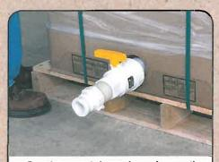
Continue to tighten the valve until the nipple gasket is compressed against the dispense gland. The valve handle should finish between the 10:00 - 2:00 position.
